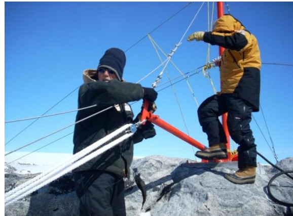
Raising the mast using the block and tackle
