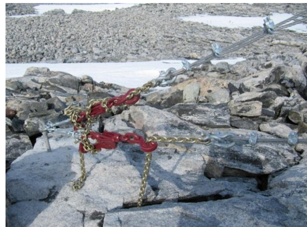
Guy wires tightened
