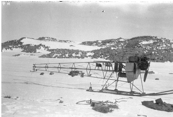
Mawsons plane at Cape Denison, ready to be used as an 'Air Tractor'. There are now 3 seats, the third being made at Cape Denison.
