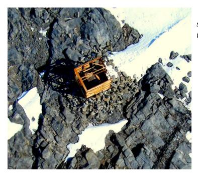
Transit hut seen from the air shows clearly how it is anchored to the rock by a pile of boulders.
