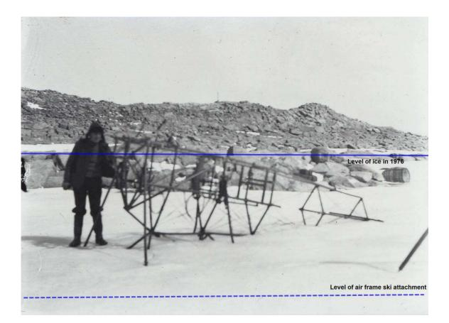
Therefore when the 1975 picture by Bob Reeves was taken, the bottom of the frame must have been about 2m below the surface. The picture from 1981 (see next section) shows exposed rocks almost up to the position of the airframe as deduced from transits. This implies that there must be a drop-off or valley in the rocks at least 2m deep just at the edge of the rocks.
