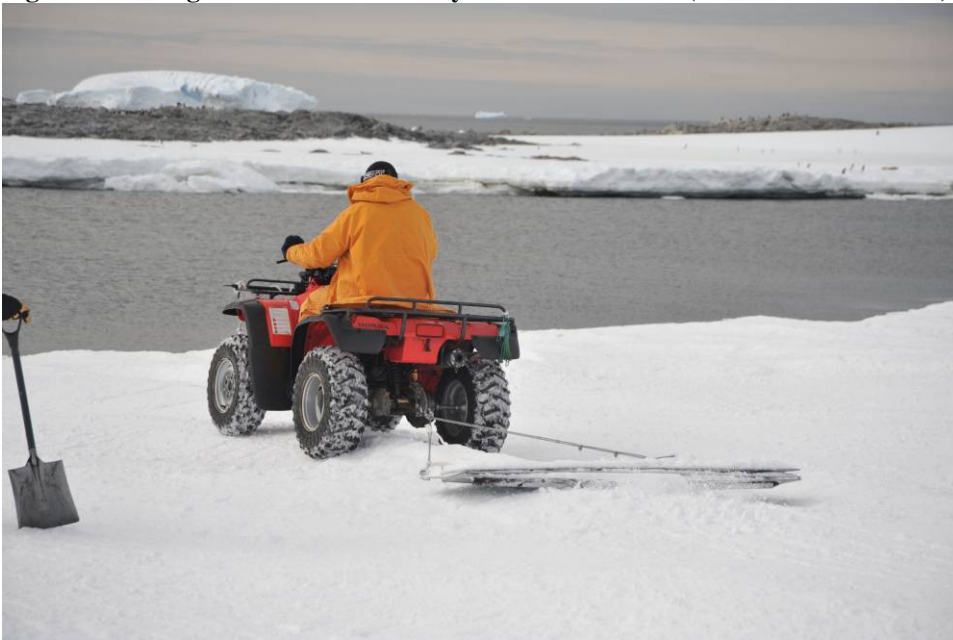
Figure 19:clearing sastrugi with a custom made cutting implement (Photo: David London)
